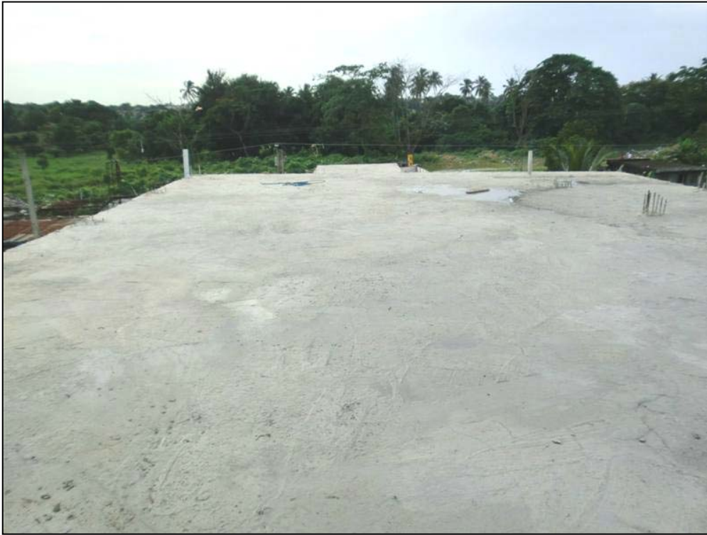
The Finished Upper Roof
