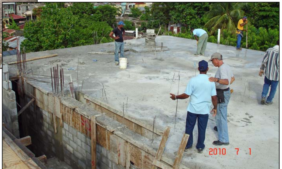
The Poured Lower Roof
