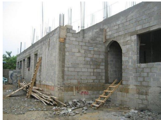
San Pedro y San Pablo with roof poured.
